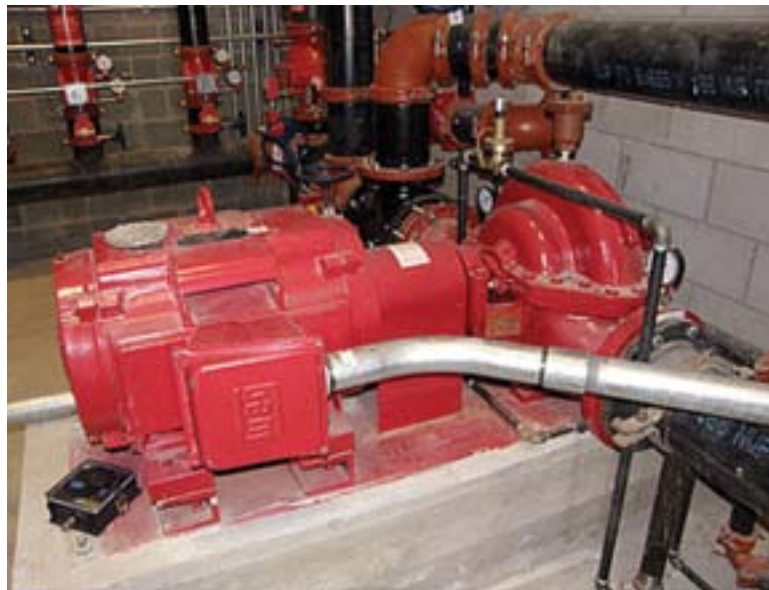
Electric horizontal split-case fire pump
