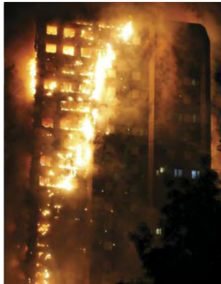
The Grenfell Tower Fire is believed to have started on the 4th storey of a 27 storey high-rise in the UK in June 2017, and ultimately spread to every storey, with tragic consequences.
