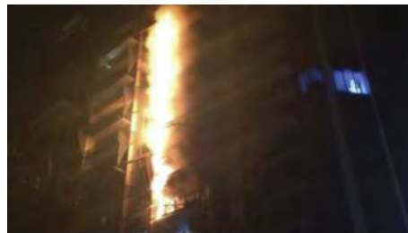
Fire raced up Dockland's Lacrosse tower in 2014 in just 15 minutes, as flammable aluminium cladding caught fire.**
